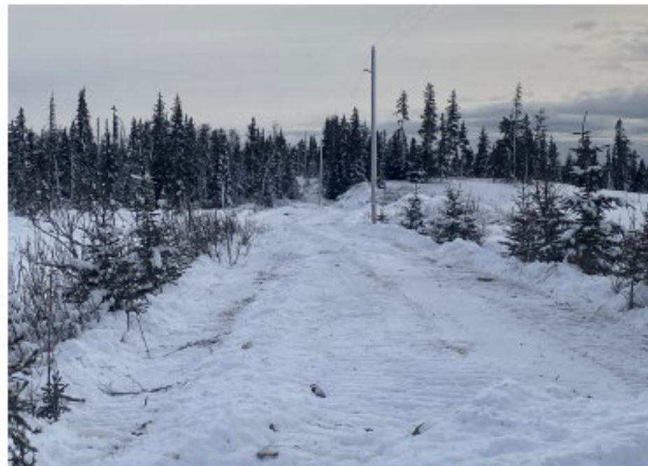
Ice road construction, Cone St. sale (Diane Campbell, 2021)
